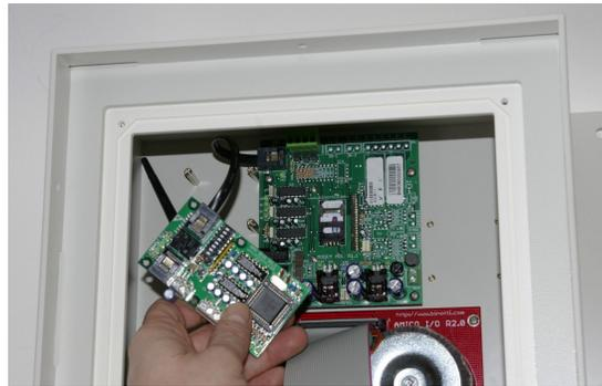
Installation of the AmiBus module (Figure 11)
